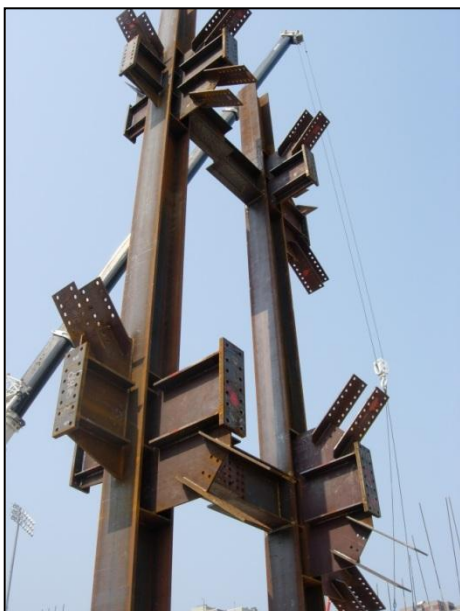
Figure 6: Connection construction photo
